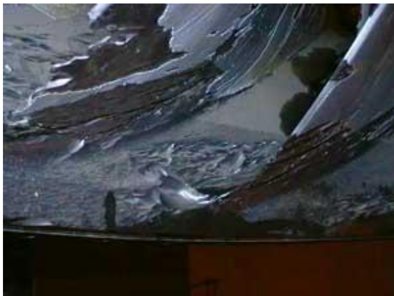
Fig. 2 Hydro-abrasive particle damage on the trailing edge of a Francis turbine [11]
